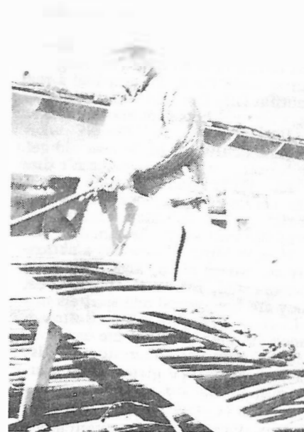
Russell putting final "U" connection on pipes before laying glass cover. Idea is similar to that used for years in Southland to heat domestic water.
